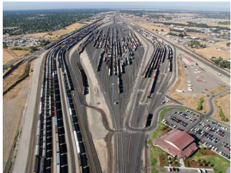
Figure 13 – UPRR JR Davis Yard
