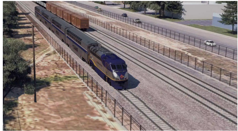
Figure 4– CCJPA Train along new Third Main Line Track
