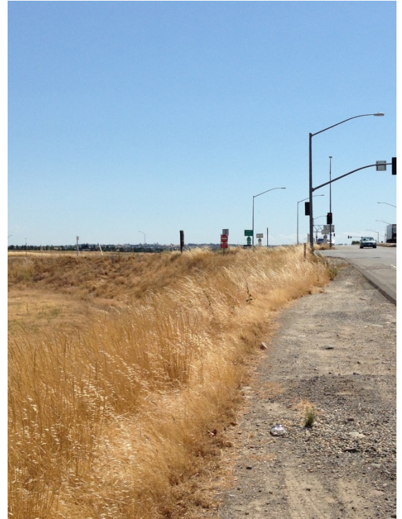
Photo 11 on-ramp at Twelve Bridges
