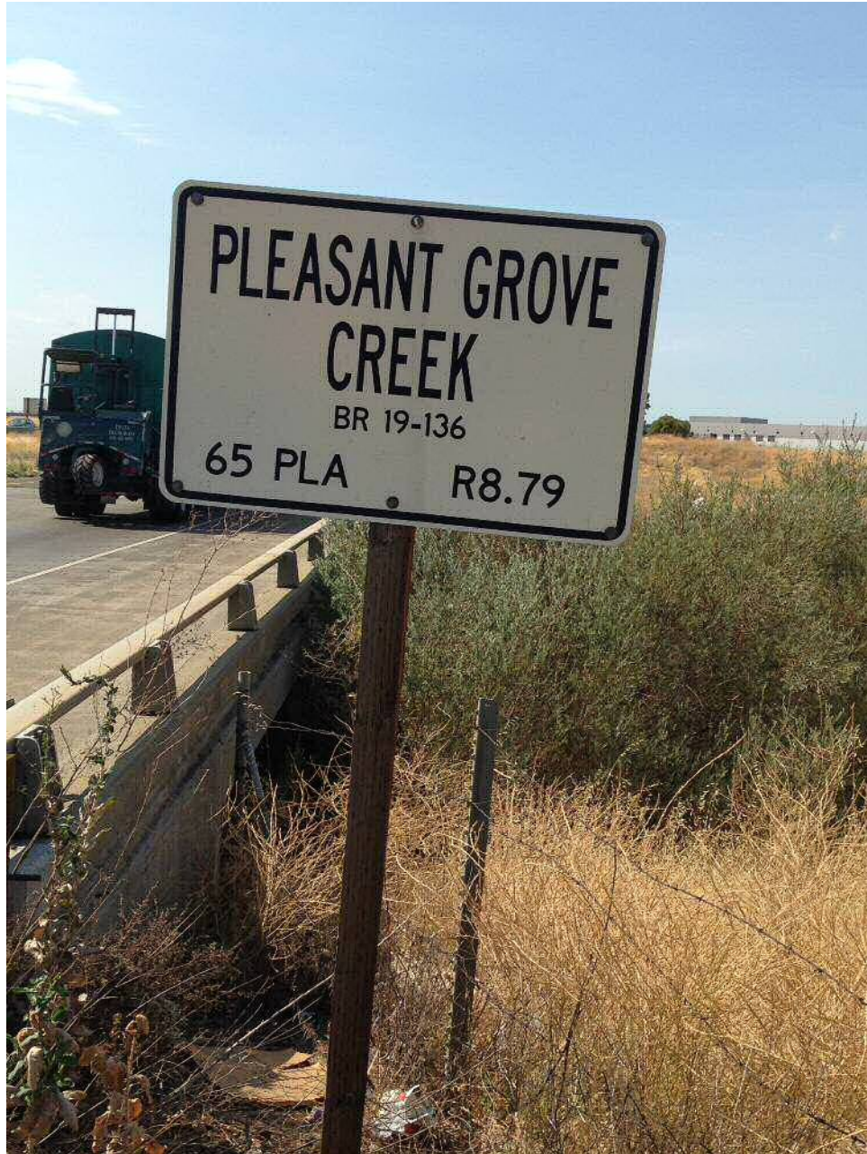
Pleasant Grove Creek Bridge
