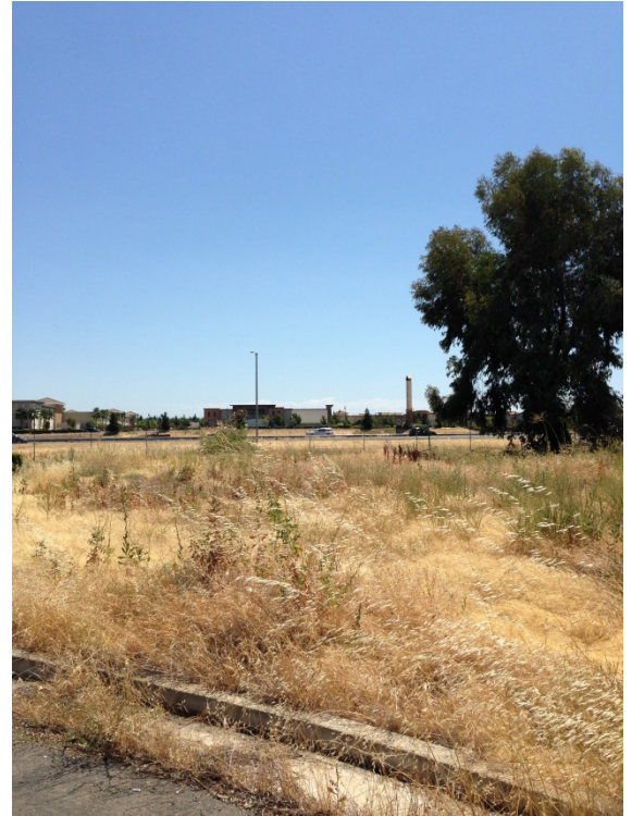
Photo 23 North of SB SR65 Blue Rock exit
