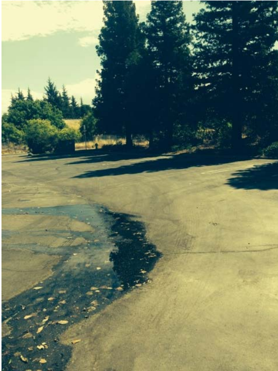
Photo 29 Drainage behind Gap, Inc.
