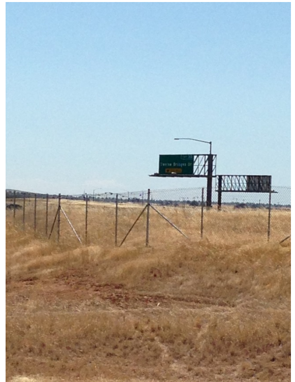
Photo 8 East of SR65 at Twelve Bridges
