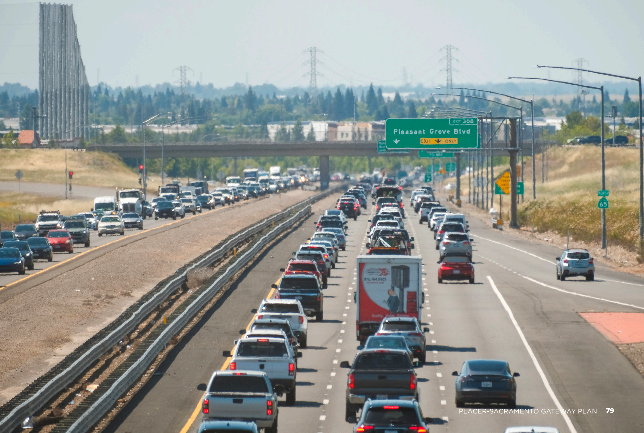
Congestion on Southbound State Route 65 Looking South from Pleasant Grove Boulevard Towards Interstate 80
